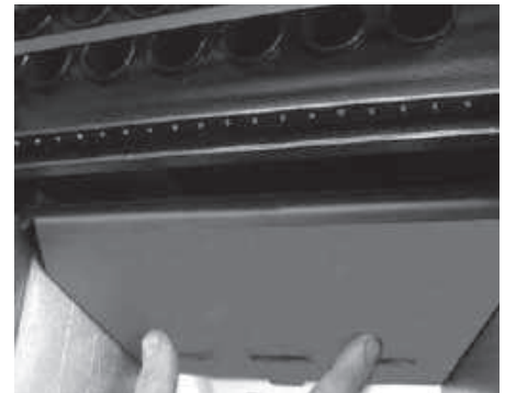
Pict. 14: Lift the fire shield
